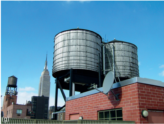
Photo 1 (a) D-type, 2 drum watertube boiler, (b) firetube boiler, (c) cooling towers, (d) chiller plant, (e) surface condenser, (f) retort cooker; (g) domestic water storage tanks, (h) hotel hot water storage vessels.
