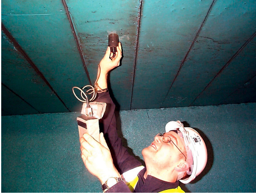
Figure 3 Electromagnetic covermeter used to locate steel reinforcement.
