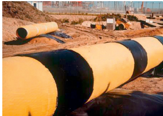
Figure 14 Moulded thermally insulated field joints.
