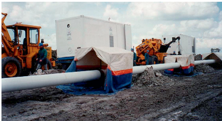
Figure 3 Typical field joint coating spread, including weatherproof shelters.
