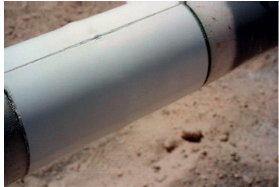
Figure 7 Coextruded polypropylene sheet in place over the field joint.
