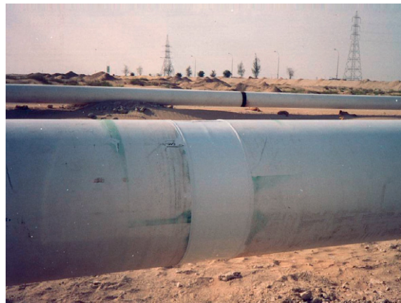
Figure 8 Final appearance after plastic welding at the horizontal and circumferential seams.
