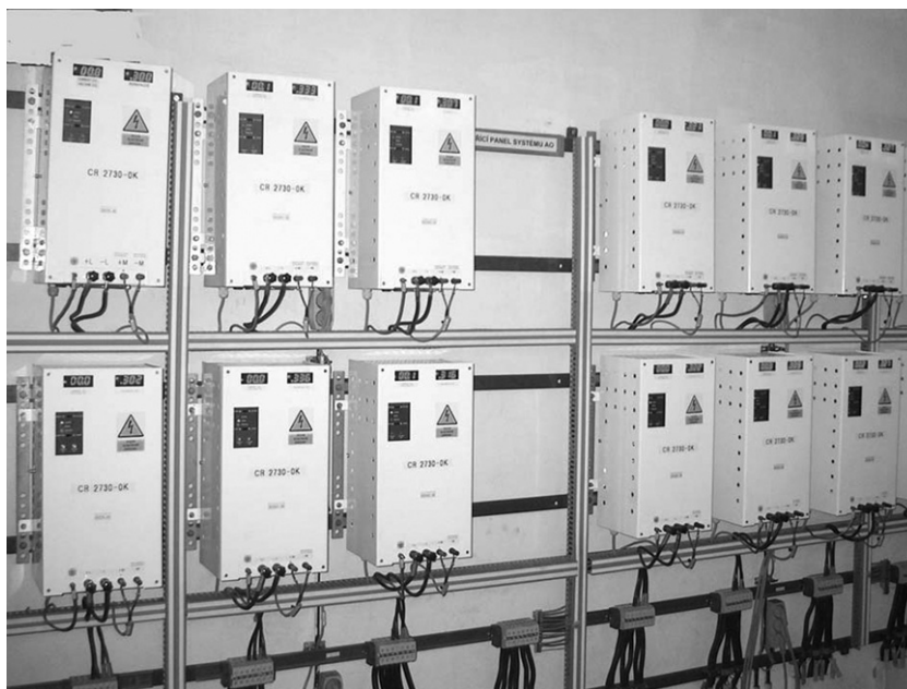
Figure 3 Main and back-up sources (potentiostats) for six anodically protected objects.
