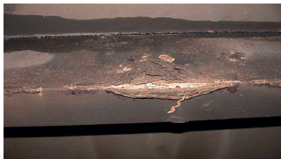
Figure 3 Rust jacking.
